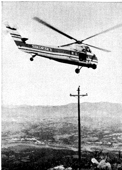
Sikorsky S-58 being used to set electric poles in difficult locations
